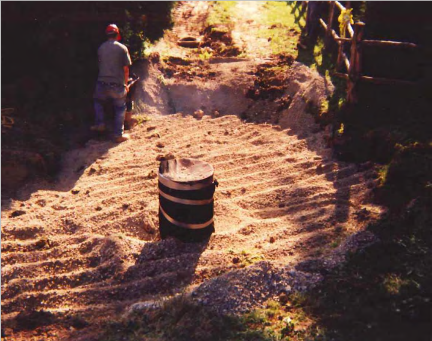
Inlet pipe with filter cloth
