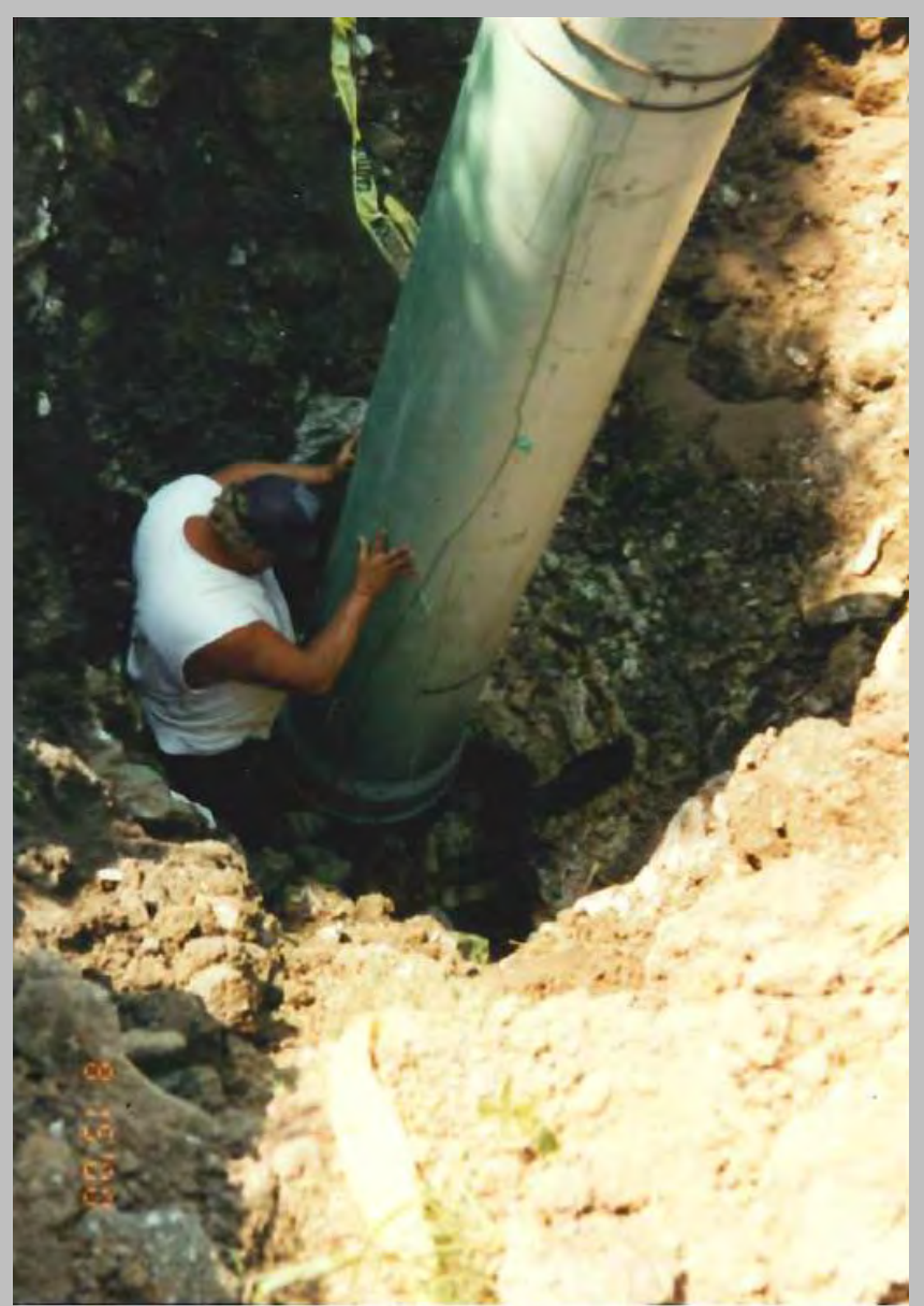
Vertical pipe being set into sinkhole swallet
