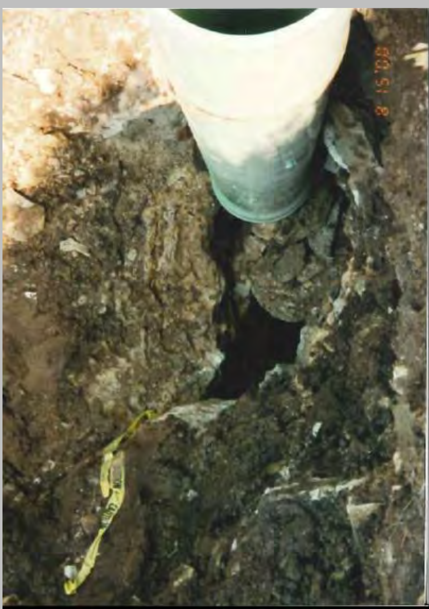
Vertical pipe being set into sinkhole swallet
