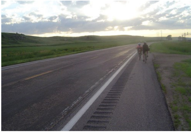
Rumble strips on the left-most edge of the shoulder maximizes the ride-able space for bicyclists.
