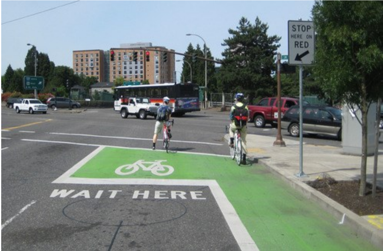
A bike box allows cyclists to wait in front of traffic, providing high visibility and ahead start over vehicle
