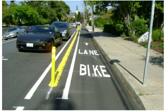
Bollards may be removed in winter to provide access to snow plow trucks
