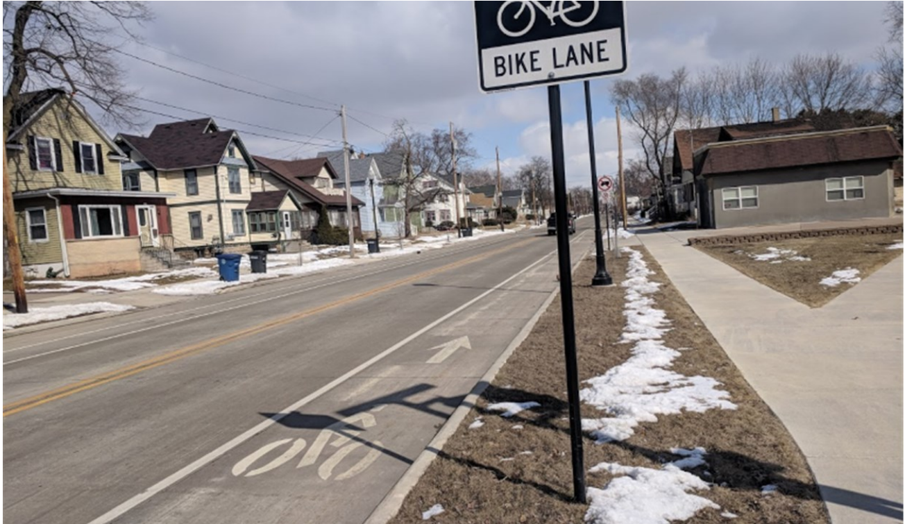
A wide solid line separates the bike lane from the roadway
