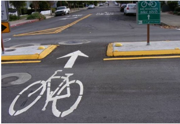
Traffic diverter used to reduce traffic
