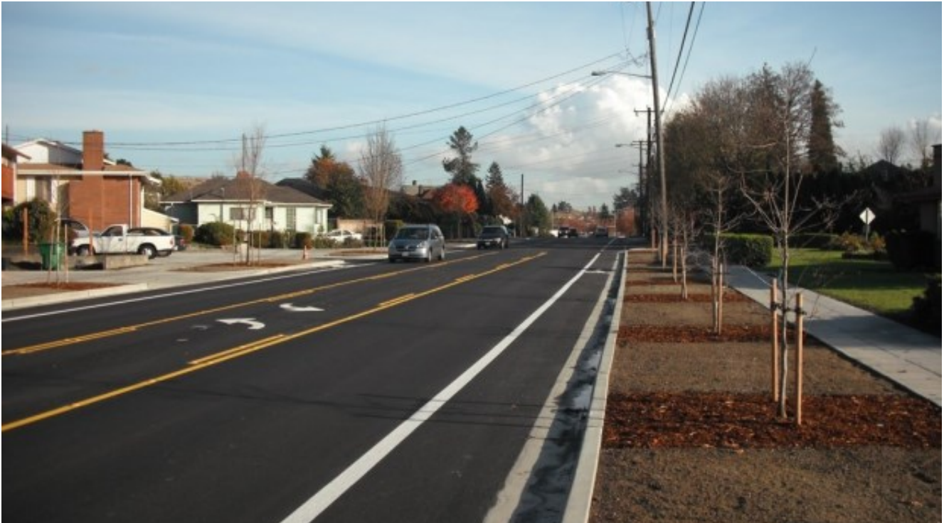
Lanes were narrowed to make way for a bike lane.
