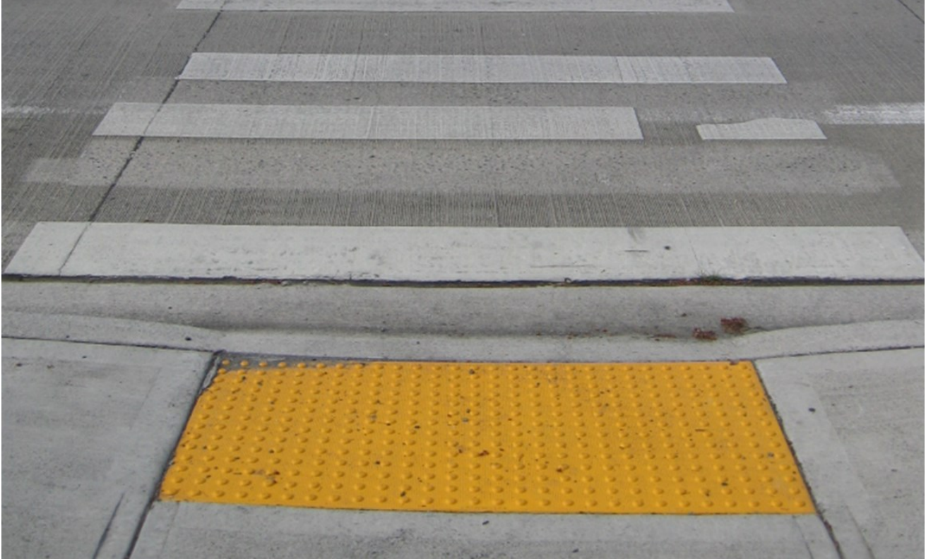
Curb ramps must include textured patterns for the visually impaired
