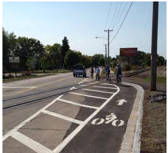
Left: Sample railroad crossing designs (from WisDOT's Bicycle Facility Design Handbook ). Above: Photo of bike lane railroad crossing on E. Newberry Street in Appleton, WI.
